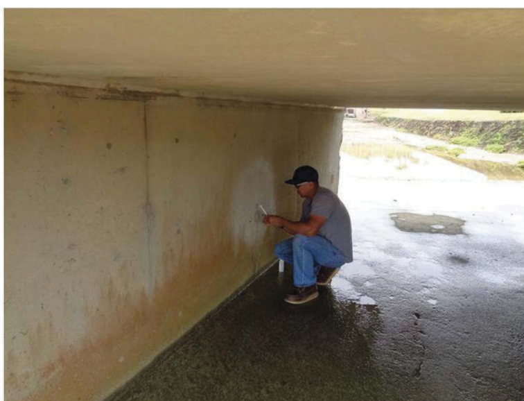
Figure 6 – Collecting rilem test tube, white area where Surtreat system applied
