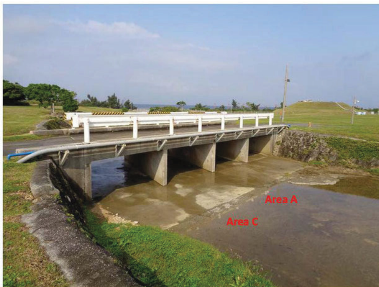
Figure 3 – View from upstream of Bridge 2 at the Kuwae Tank Farm, Kadena AFB, 2016
