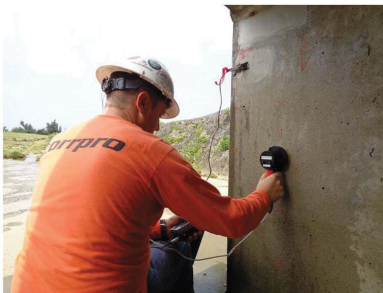
Figure 5 – Measuring corrosion rate
