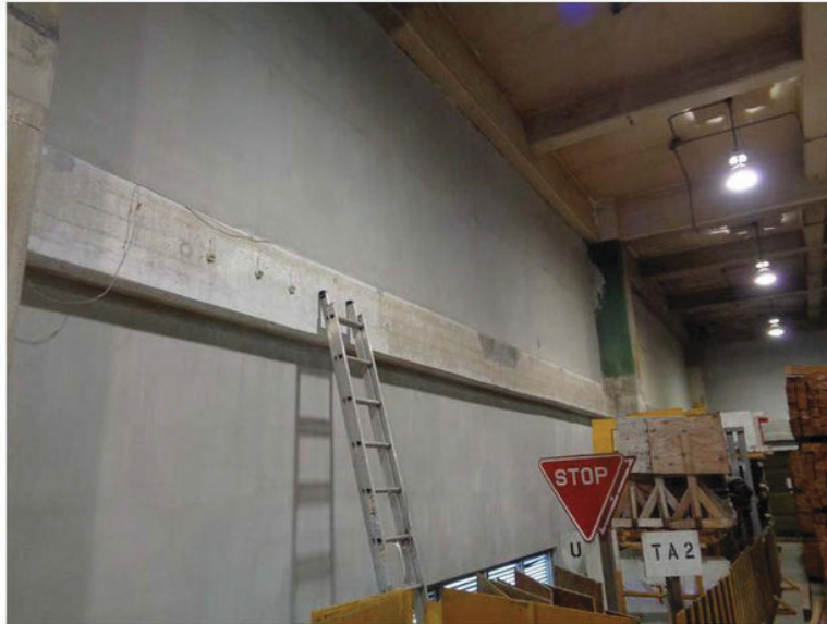
Figure 11 – Rilem test tubes placed on section 1 ring girder.
